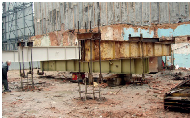
Figure 6. Static tests of piles using hydraulic jacks
